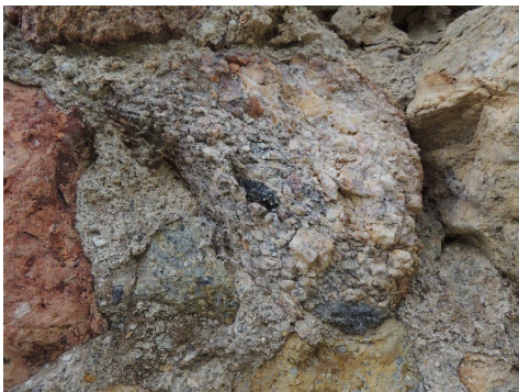
Fig. 8- Masonry ashlars in microconglomerate from the "Anageniti minute Formation"(photo by F. Fratini)
