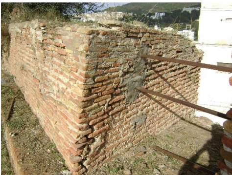
Fig. 4- Exterior facing (Maya Akouche, 2023)
