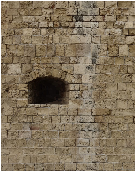
Fig. 7- A detail from the photogrammetry of the north-eastern front (the Authors).
