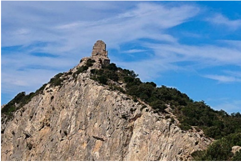
Fig. 1- Image of the Capo d'Uomo Tower from the north-west.
